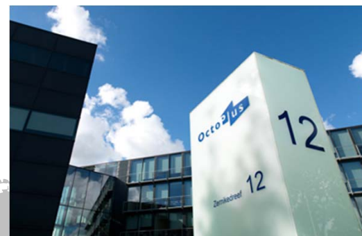
Octopus Technology Development Centre Leiden, Netherlands
