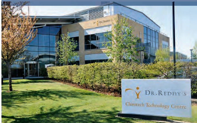
THE EXPANDED CHIROTECH TECHNOLOGY CENTRE IN CAMBRIDGE, UK
