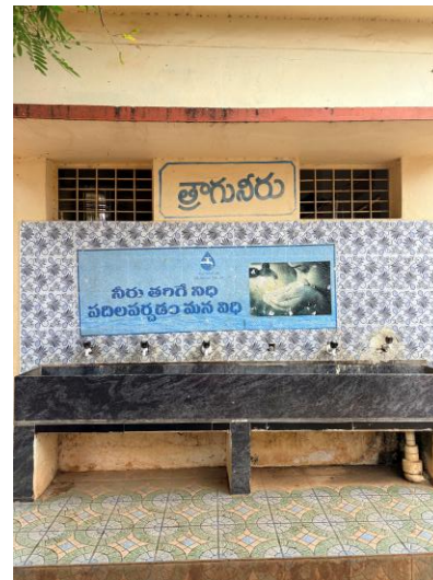
Renovated drinking water station
